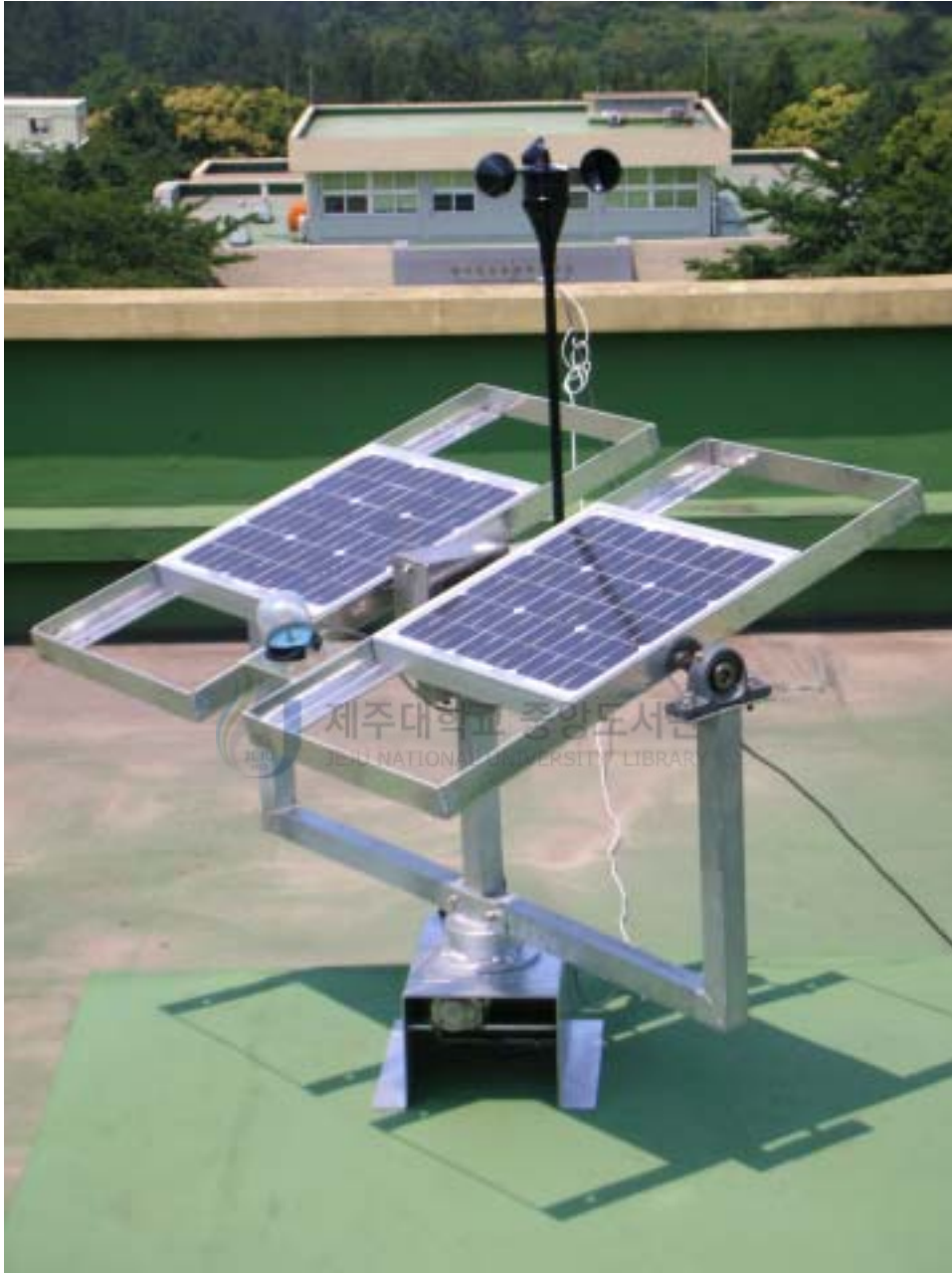
Fig. 3-7 Photograph of solar position tracking system
