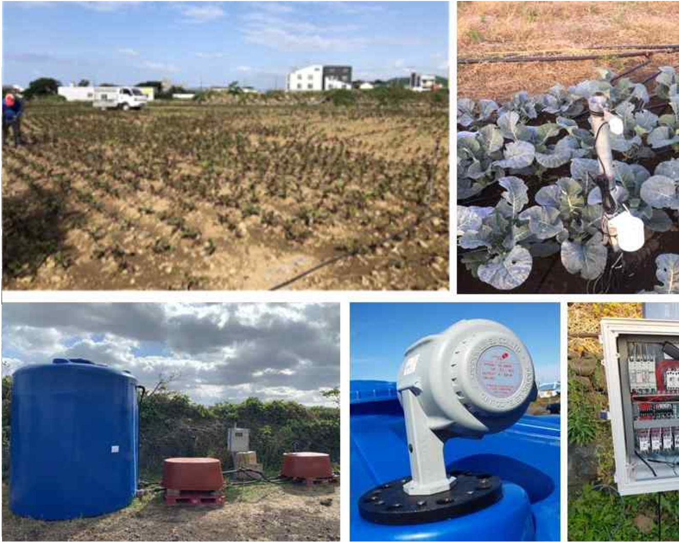
Fig. 19 Construction of irrigation tanks and pumping pumps
