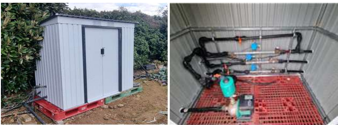
Fig. 20 Construction of irrigation pump rooms and pump facilities
