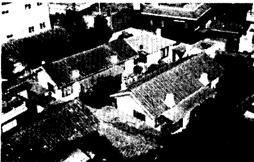
Fig. 3 An outside view of Welfare House(Located at Samdo-1dong)
